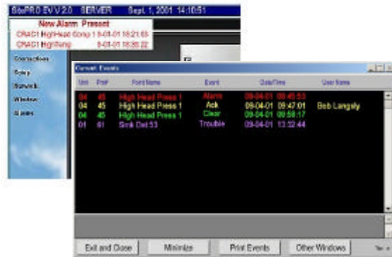
Active Alarm and Current Event Windows
